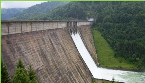
Hydropower Plant Bicaz
